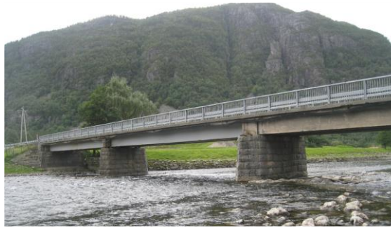
Figure 1. Considered road bridge
