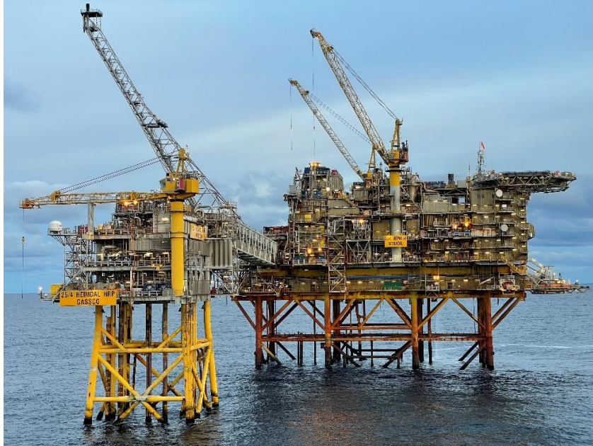
Figure 1. Heimdal platform, typical offshore jacket structure
